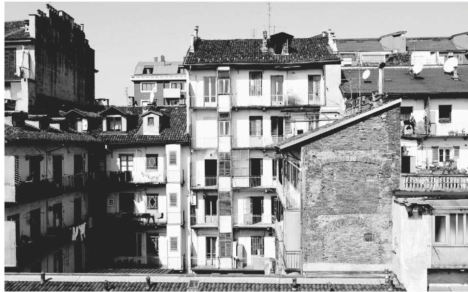
Figure 4. Internal view of the courtyard of the Giulio34 project building. Source: photograph taken during the carpentry workshop by Carlos Lapo Procel.
